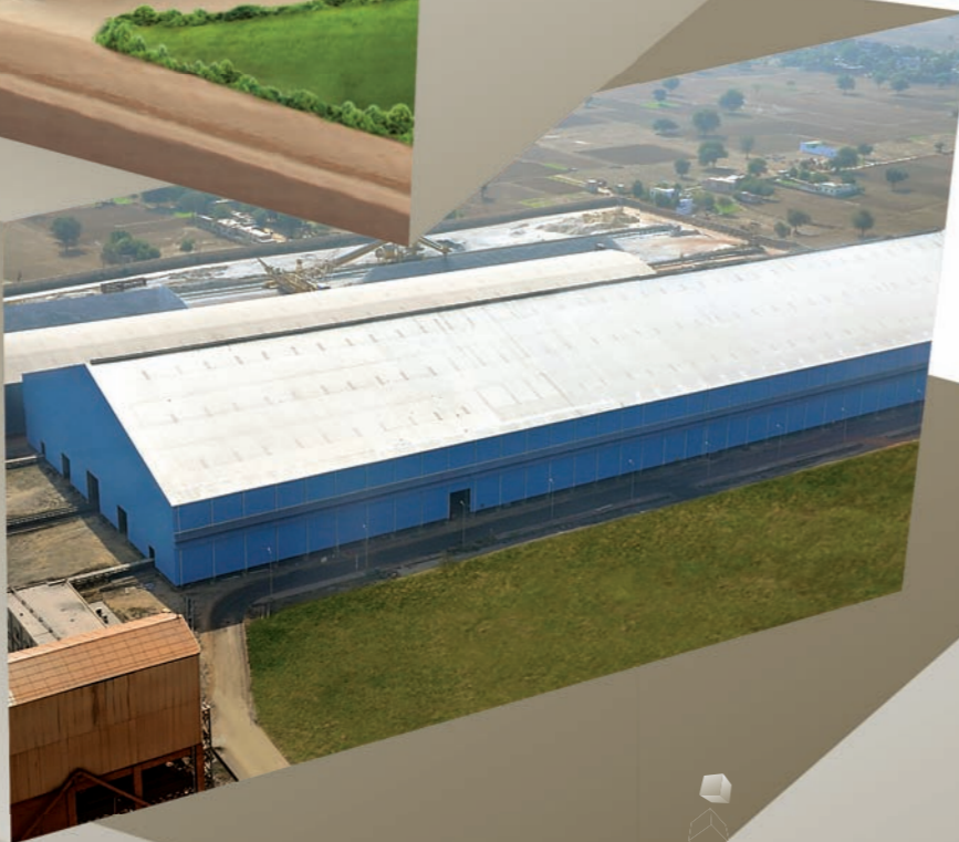
99m Clear Span Building for UltraTech Cement Ltd., Kotputli, Rajasthan
