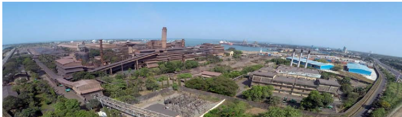
[Aerial view of Pellet Plant at Mangaluru]
