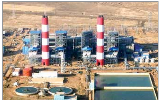
4x125 MW Kosti Thermal Power Plant, Sudan
