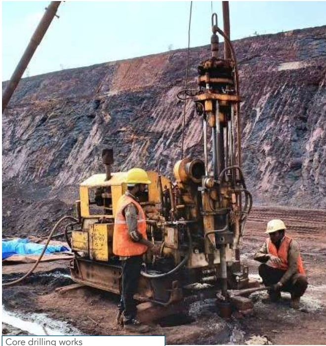
Core drilling works
