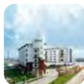
Fortis Hospital Shalimar Bagh, Delhi
