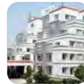
Fortis Hospital Vasant Kunj, Delhi
